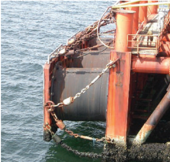
Fig. 1 Circular shaped buckling fender: 3000H
