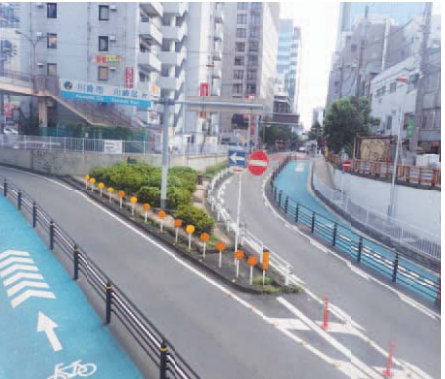
Installation of bicycle lanes in front of stations
