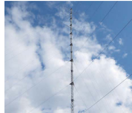
Wind condition observation tower
