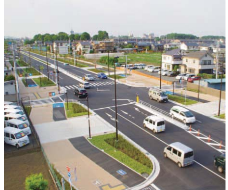
Maintenance of primary local roads (removal of utility poles, promote barrier-free)
