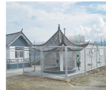
Planning/construction of rural wastewater treatment facilities (China)
